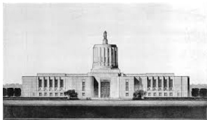
WYNNE JONES, OREGON STATE CAPITOL BUILDING, SALEM, OREGON Photo: Oregon Department of Parks, Recreation and Heritage
